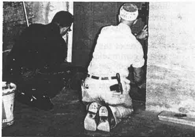
Figure 14. Seal structure to be fumigated
