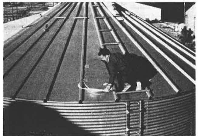
Figure 8. Sealing openings of storage bin
