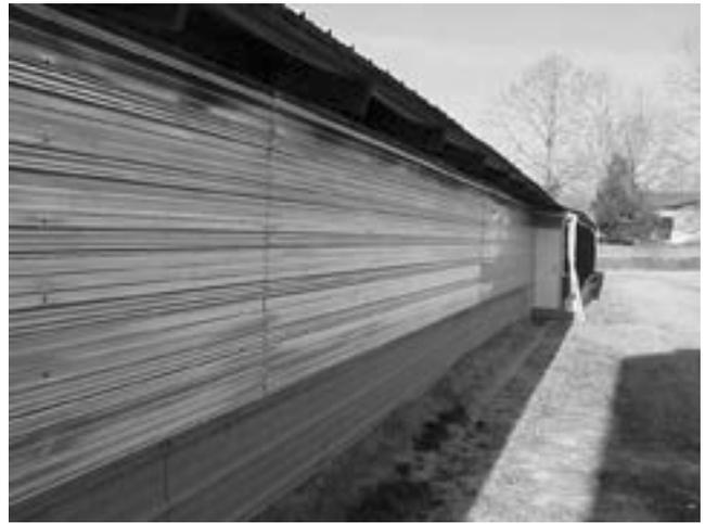
A common solid sidewall retrofit is to nail 2-inch lumber over the curtain opening, as shown here at left. It is important to put a good vapor barrier such as 30# felt on the back side of the lumber before nailing the tin on the outside. Putting fiberglass or batt insulation into the wall in this type of construction is difficult. The photo at right shows how this type of construction might look from the outside. Note the new tin over where the curtain opening used to be.
