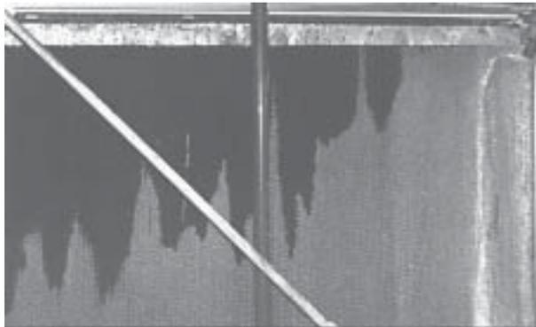
The distribution header at the top right portion of this cooling pad is clogged. Holes in header pipes must be kept clean or parts of the pad will receive no water. Any dry area on a cooling pad (recirculating or spray-on) will allow hot air to enter the house, canceling the effect of evaporative cooling. Pads must be kept thoroughly wet.
