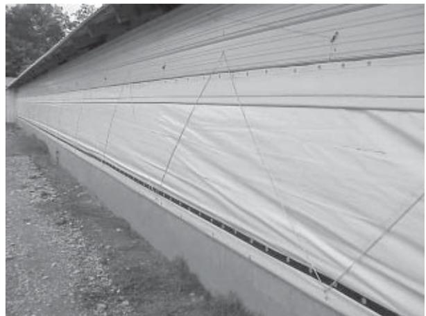
Curtain flaps such as shown here are extremely important to block air leaking around the curtain. Curtain leaks allow large amounts of hot outside air to enter the house and at the same time steal from airflow through the tunnel air inlets and through the cooling pads (if used).
