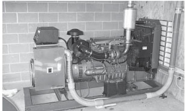
Standby generators are critically important for modern tunnel-ventilated broiler houses, since power failure can cause catastrophic losses within minutes. To insure they are ready and available, generator sets should be operated on automatic transfer switches, serviced regularly, and test-run for 30 minutes once a week.
