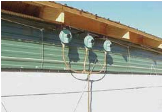
The trunk line from the gas tank and first stage regulator branches to serve three second stage regulators, which take gas at 10 psi and reduce the pressure to approximately 11-13 inches of water column. Second stage regulators should be located outside the house.
