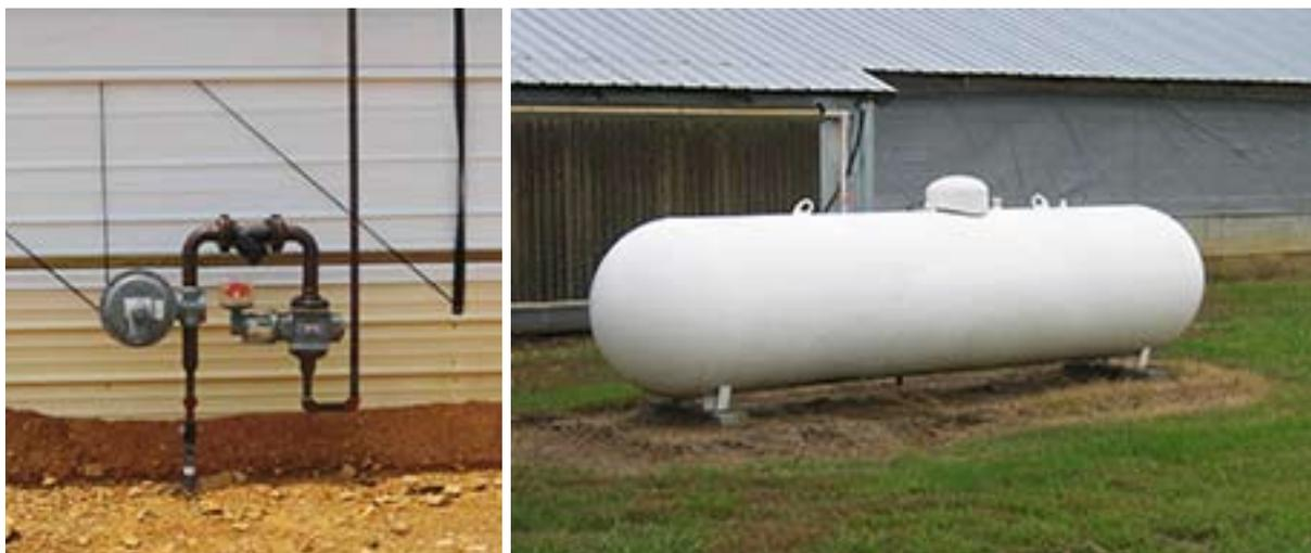
Conversion from propane to natural gas is typically advantageous in areas where natural gas lines are located close enough to the farm. The conversion process involves changes or modification of equipment, such as trading propane tanks for natural gas meters, shown at left.
