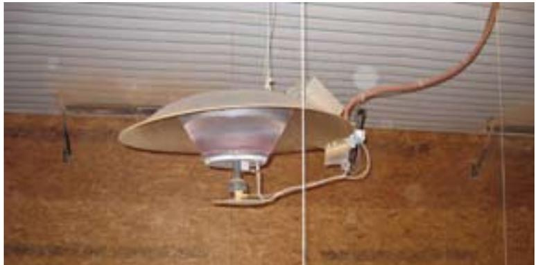
less than half the heat content of propane, and the old timers were not delivering the correct volume of natural gas to the appliance. It takes approximately 2.5 times the volume of natural gas to produce the same amount of heat as it does propane. Burning one cubic foot of natural gas produces approximately 1,012 BTU's of heat while burning one cubic foot of propane produces 2,520 BTU's of heat.
