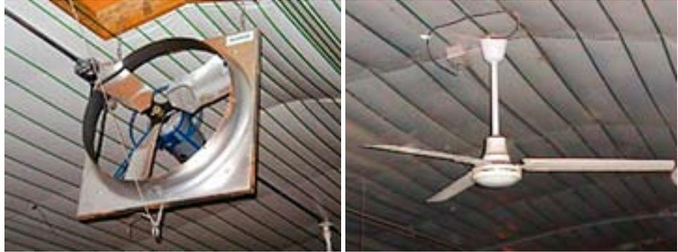
**Stir fans can significantly cut fuel use and improve bird performance in both old and new houses. Many variations exist. Axial fans are most recommended for low ceiling houses. Paddle fans are used successfully in high ceiling houses. Newer houses can typically get around 10% in fuel savings; older houses may see as much as 25% savings.**
