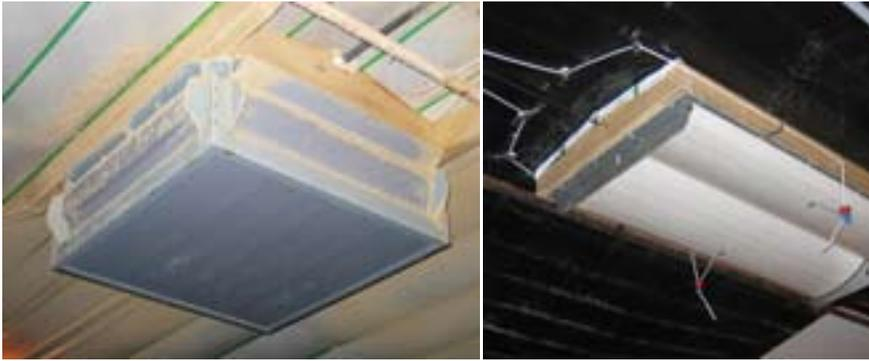
Using attic inlets to provide pre-heated bird chamber air can save as much of 20% of yearly gas costs. Photos show a gravity-type attic inlet (at left) and a controller-actuated inlet (at right). Houses must be tight and attic inlets managed properly to avoid allowing moist, warm in-house air to get into the attic.
