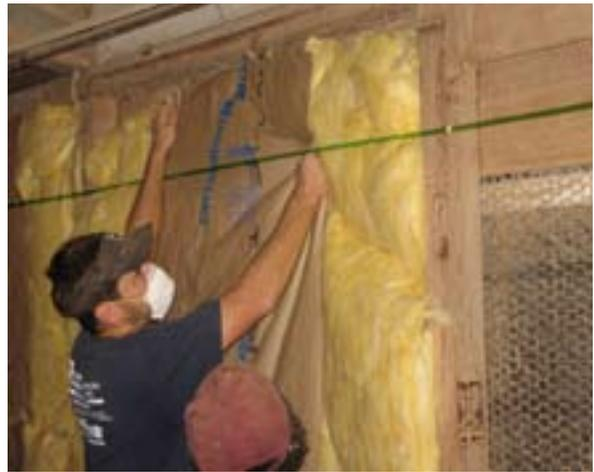
**There are many ways to insulate sidewalls. One of the best methods is to add a 3-inch fiberglass batt between existing posts, as shown in this photo. Wall R-value increases from R-1 to R-11, drastically reducing the amount of heat lost through sidewalls.**
