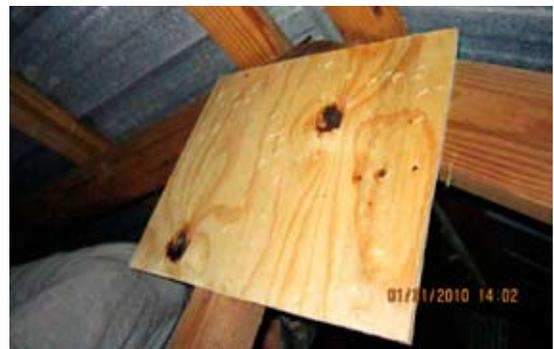
Photo above shows an acceptable truss repair in progress. The plate is 3/8-inch plywood of significant size being applied with numerous fasteners on each truss member. This repair will be complete when a matching plate is similarly applied to the other side.
