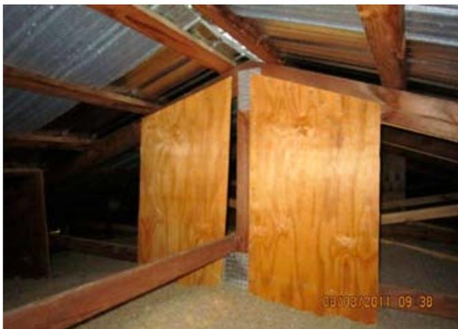
Photo at left shows an acceptable plating repair of a truss whose center metal truss plates had come loose. Numerous screws were used instead of nails in the plywood plates. A matching plate on the other side makes this truss as strong or stronger than it was prior to the damage. However, these large plates do restrict attic access for future inspection.
