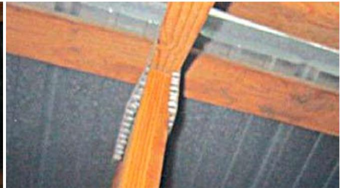
The truss plates on these trusses are in the first stage of failure, beginning to pull out and allow the trusses to deform. Neither of these trusses showed any sign of a problem from the outside of the house. Only through close attic inspection can this be found. This may be the result of a storm event or normal aging.
