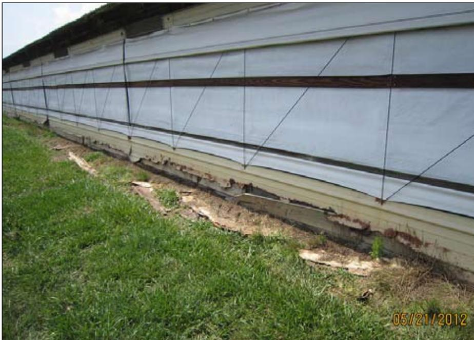
**Metal along the lower sidewall of poultry houses is exposed to many corrosive forces. If not addressed, this corrosion can become severe, causing multiple problems. Air leakage is the most common detrimental effect. Vermin entry and compromised structural integrity can occur in the worst cases.**
