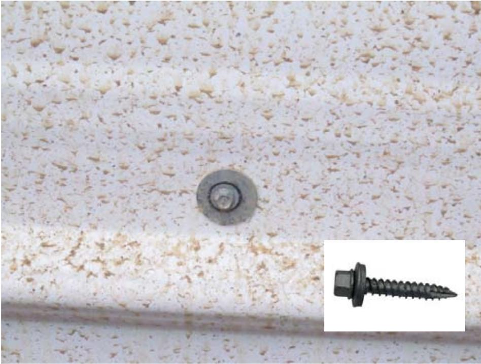
**Adding a common quarter-inch flat washer, larger than the neoprene washers that come with a typical 1-inch roofing screw, provides an additional backer that helps hold the PVC panel in place while reducing chance of potential problems with expansion/contraction down the road.**
