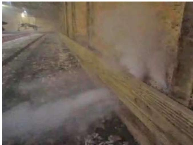
**As shown in this smoke test photo, when using negative pressure to ventilate in the winter, damaged sidewalls allow streams of cold, damp air to flow directly onto the litter at chick level. This causes a multitude of problems. Wet litter, chilled chicks and increased fuel usage to combat these are the obvious. Increased difficulties ventilating such houses will impact overall flock performance, as well.**
