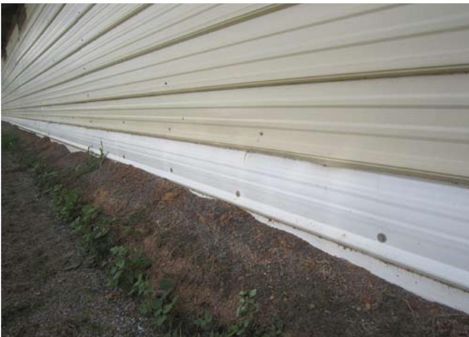
**After three years of field trials, the PVC panel repaired houses still look good and have maintained their tightness with no additional maintenance. The panels remain tightly installed to the lumber beneath with no signs of cracking or fasteners loosening. This house is ready for several more years of service.**
