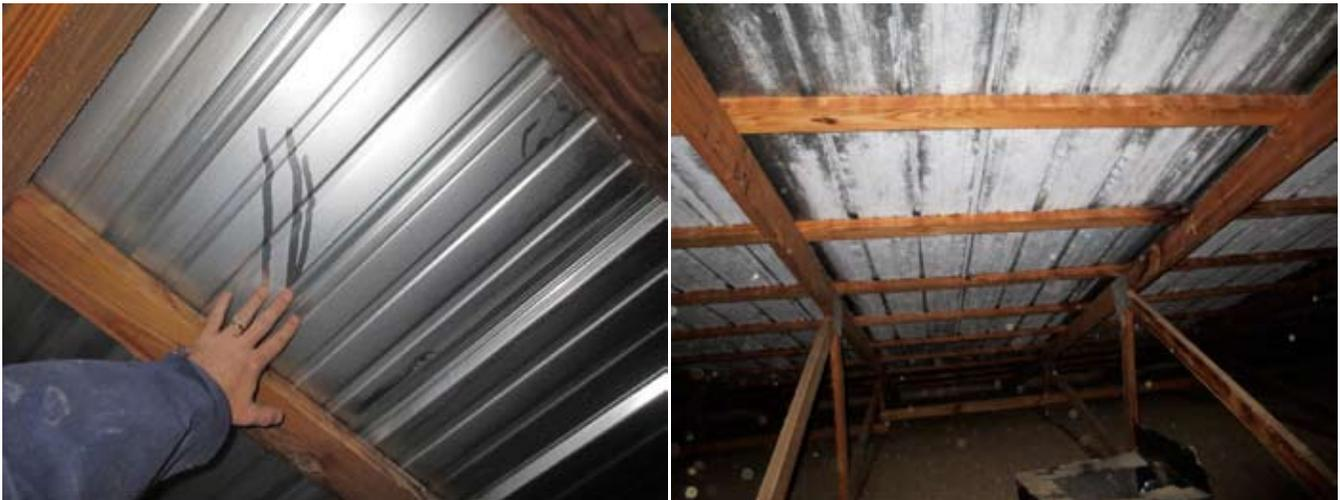
**Condensation on Roofing and Attic Lumber Can Threaten House Structural Integrity:**
