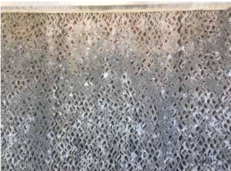
**These pads have substantial mineral and dust buildup collected on the outside surface that will drastically reduce airflow during tunnel ventilation. Cleaning dirty pads can be another opportunity to gain 50 fpm or more in wind-speed – in addition to getting better cooling.**
