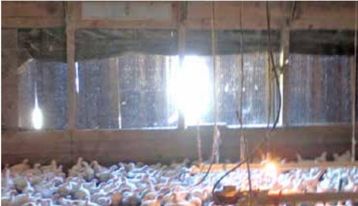
**This photo of an operating pad system with a section of pads missing shows one of the worst-case ways hot air is too often allowed to bypass the cooling system. Outside air that bypasses the pads is not only uncooled, it enters the house much faster than air that flows through the pads. Spring is the time to make sure all air enters through the pads this summer and birds get the cooling they need.**
