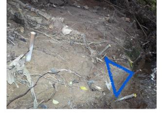
hammer to make your pilot hole approximately 2 feet into the bank. Dead blow hammer heads may become damaged with repeated forces applied to rebar. Do not insert the rebar so far into the bank that you cannot pull it out! Remove the rebar from the streambank.
