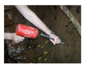
and live stake should be made at a 90° angle to streambank. Use a dead blow or sledge
