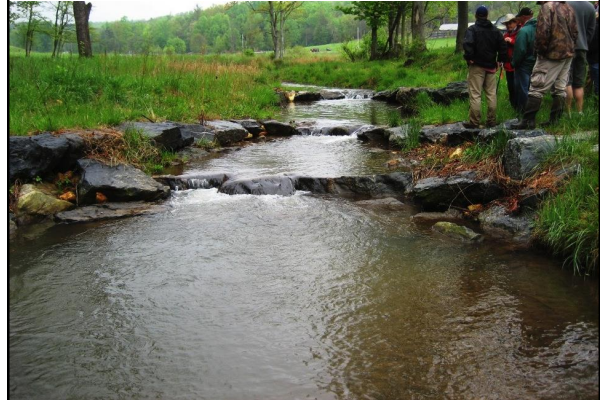
Double-Drop Boulder Cross Vane
