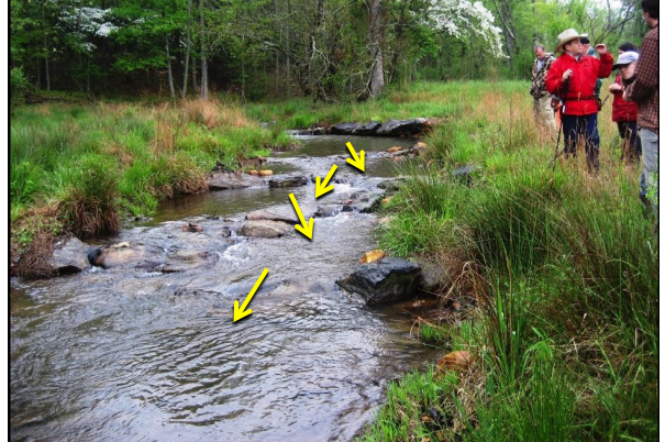
Constructed Riffle (Rock & Roll)
