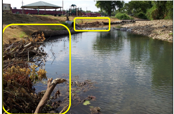
Toe Wood for bank protection, roughness, habitat
