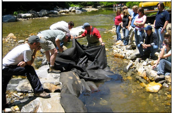
Geotextile Curtain to Prevent Piping
