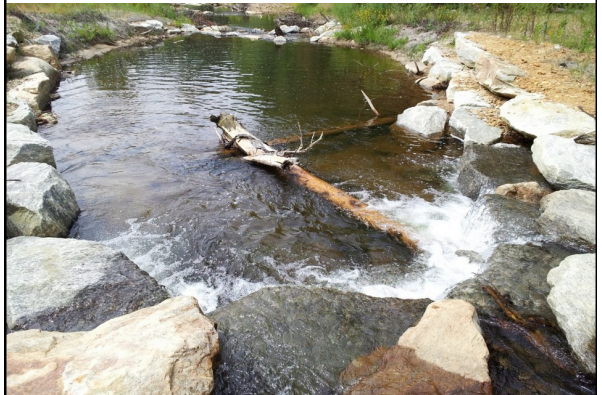
Cross Vane (logs embedded)
