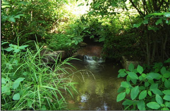
Culvert with Buried Bottom: 2011
