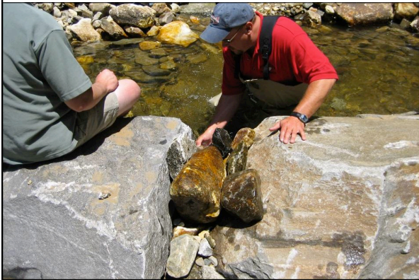
Chinking Boulders to Prevent Piping
