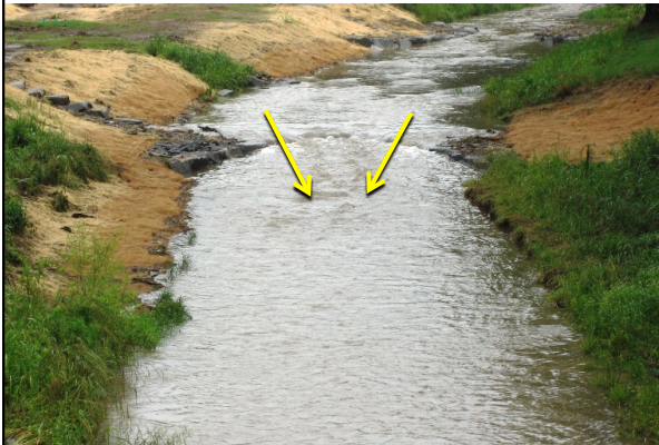
Boulder Cross Vane: Grade Control
