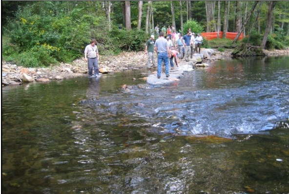
Boulder J-Hook Vane: Scour Pool
