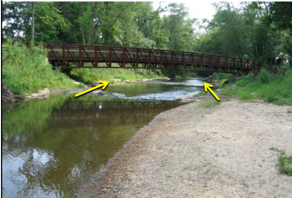
Offset Boulder Cross Vane at a Bridge
