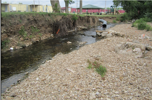
Existing Condition: Stormwater outfall pipe
