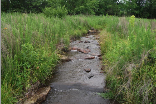
Riffle with Embedded Logs
