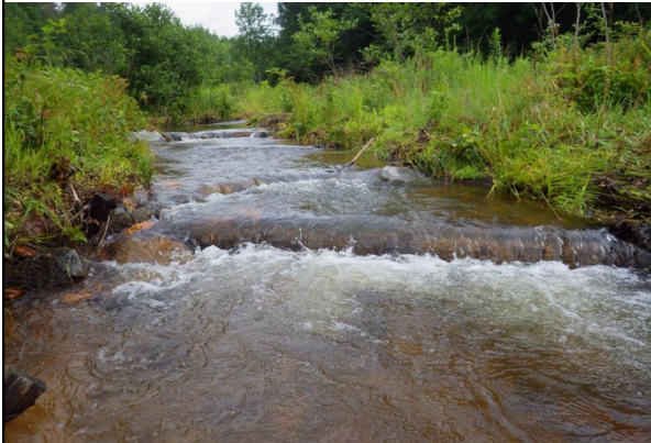
Riffle with Log Rollers
