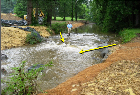
Double-Drop Offset Boulder Cross Vane
