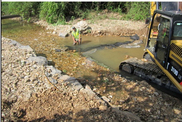
Log J-Hook Vane with Boulder sill hook & geotextile
