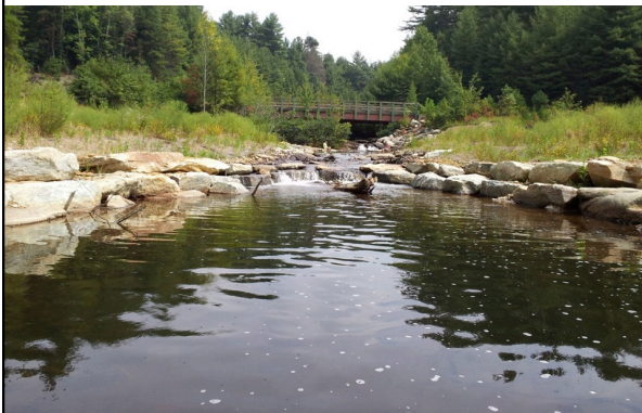
Cross Vane (logs embedded)
