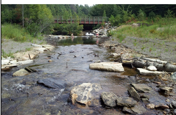
Constructed Riffle with Embedded Wood
