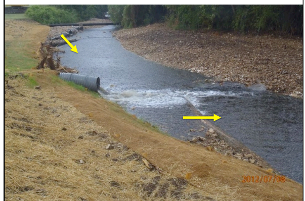
Storm Flow: Flow direction + Bank protection
