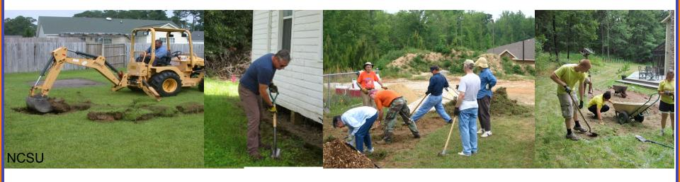
Excavation Depth = Ponding Depth (3" to 6") + Mulch Depth (3")
