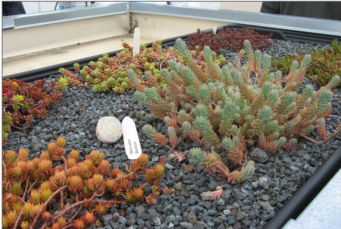
Figure 10.2. Examples of green roof vegetation at the University of Alabama at Birmingham, Birmingham, AL.
