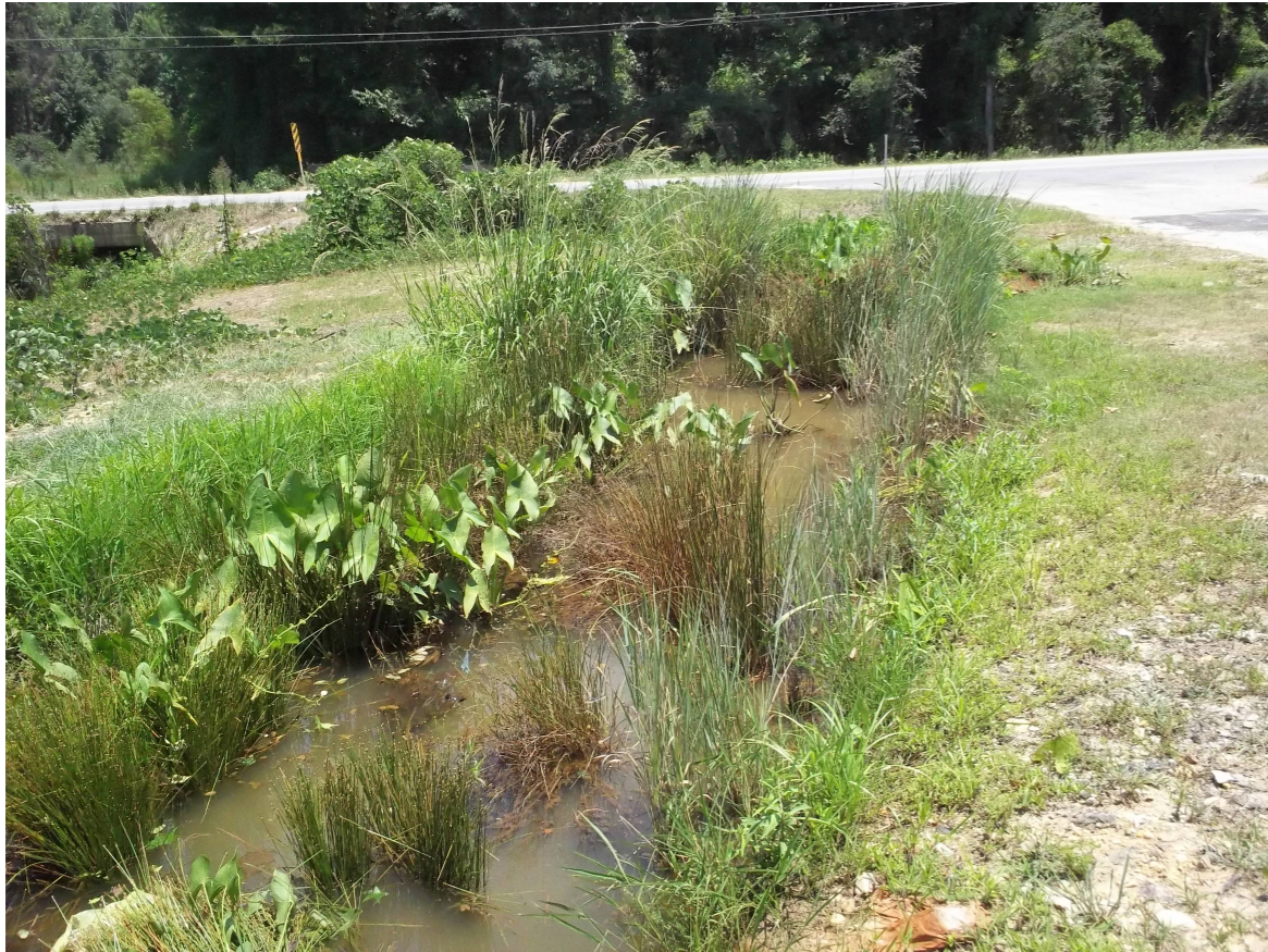
Figure D.12. Aquatic plants in a wet swale, Auburn, AL.
