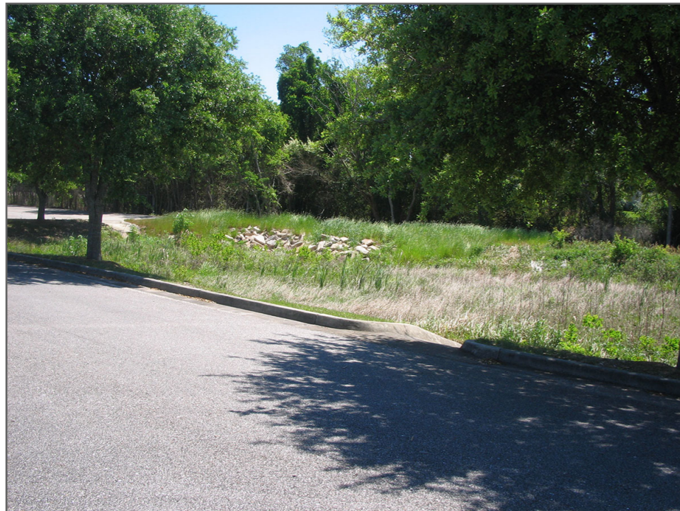
Figure 13.3. Curb cut at Hank Aaron Stadium, Mobile, AL.
