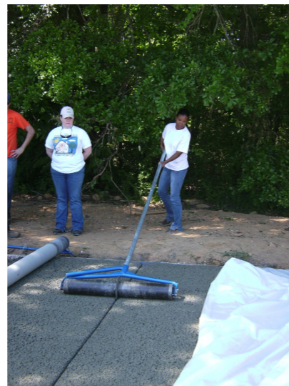
Figure 6.15. “Pizza cutter” joint tool at Duck Samford Park, Auburn, AL. (Photo courtesy of Michael Hein.)
