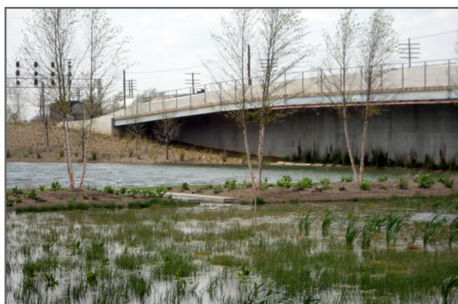
Figures 4.1. and 4.2. Bioretention in Railroad Park, Birmingham, AL.
