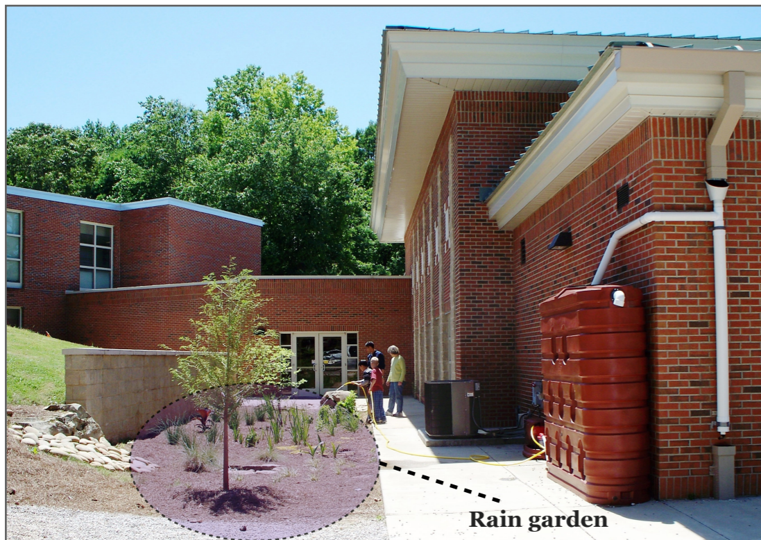
Figure 9.4. Rainwater is harvested and used to irrigate a rain garden during plant establishment at Cary Woods Elementary School, Auburn, AL.
