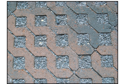
Figure 6.5. Concrete grid pavers.
