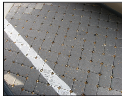
Figure 6.4. Permeable interlocking concrete pavers.
