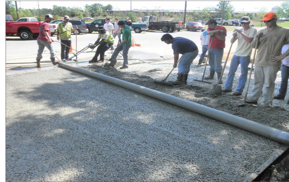
Figure 6.12. Strike-off and compression at Duck Samford Park, Auburn, AL. (Photo courtesy of Michael Hein.)
