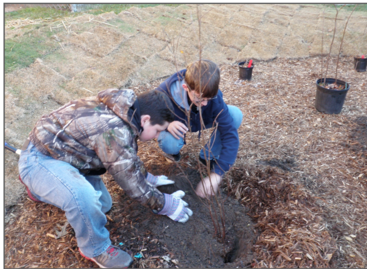
Figure D.2. Students install plants in bioretention area, Phenix City, AL.
