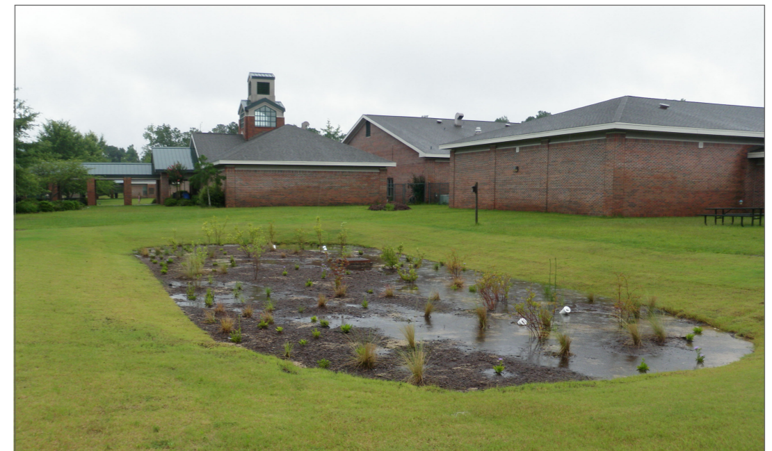
Figure 4.12. BRC three months post-installation, East Smiths Station Elementary School, Smiths Station, AL.
