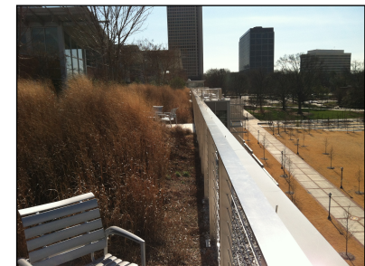
Green Roof & Cistern - GT Campus
