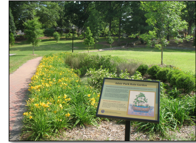
Bioretention - Adair Park
