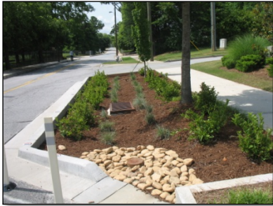
Bioretention - Curb Extension
