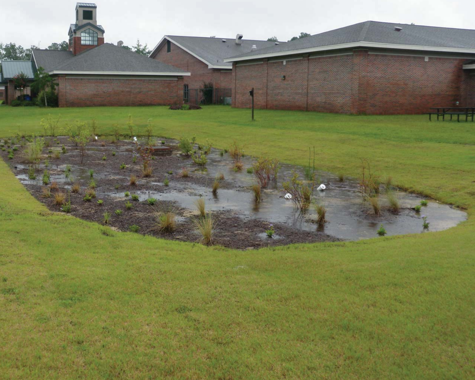
Bioretention cell 3 months post installation, East Smiths Station Elementary School; Smiths Station, AL
