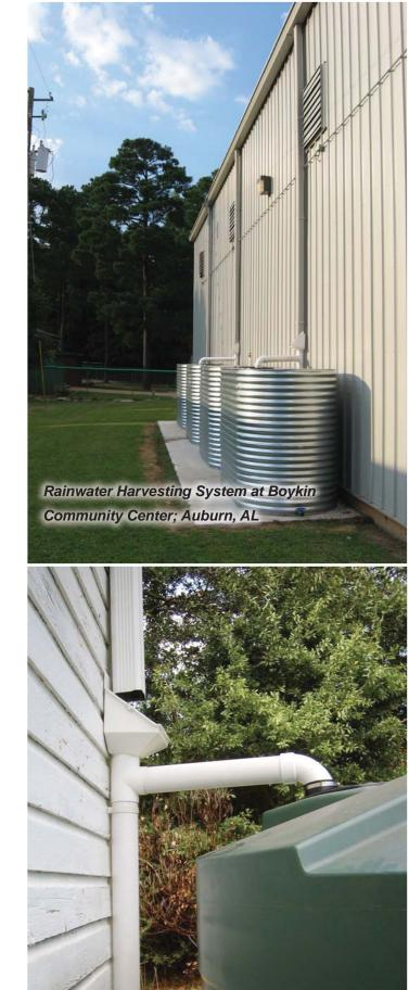
Rainhead and First Flush Diverter system;
