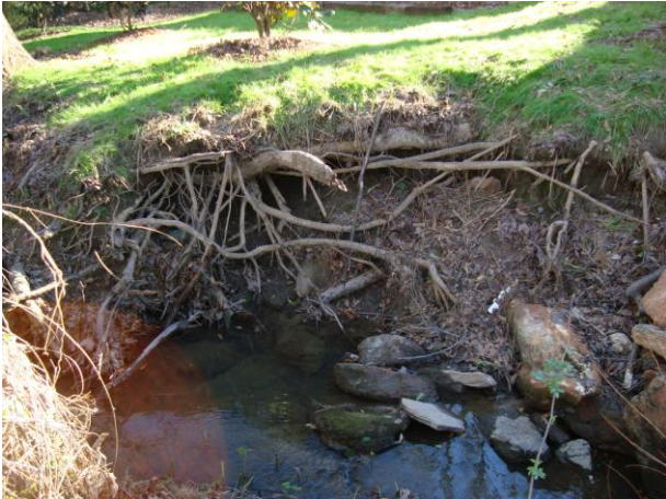
Typical erosion along stream bend, Auburn, Alabama.
