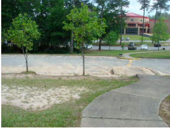
Figure 14. Sediment Deposits from High Velocity Runoff Volumes on CHS Campus.
