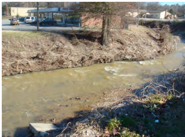
Figure 1. Mill Creek Stream Crossing at Crawford Rd. in Phenix City, AL.
