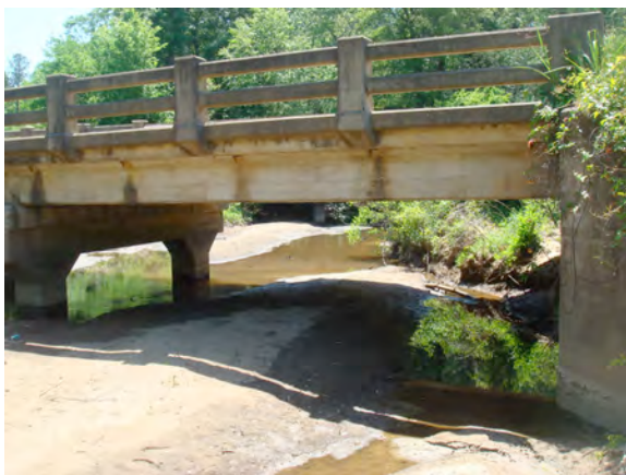
Figure 10. Mid-Channel and Lateral Bars Downstream of Construction Sites on Mill Creek.
