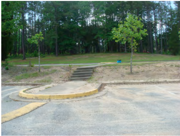
Figure 16. Severe Erosion and Subsequent Sedimentation at CHS Campus.
