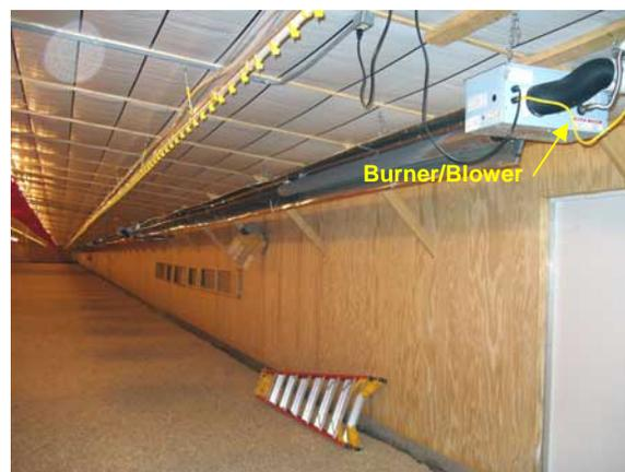
**A radiant tube heater positioned at the top of the sidewall. This installation can be used successfully with whole house brooding.**
