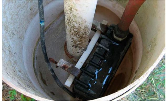
Recirculating pad cooling systems save on water costs by re-using water. However, to maintain efficient cooling, system water should be dumped and replenished as needed, usually on a weekly basis. Dirty water, as seen in sump at left, leaves all its dirt on the pad as the water evaporates, reducing the system cooling. Photo at right shows clear water in a well-maintained system.
