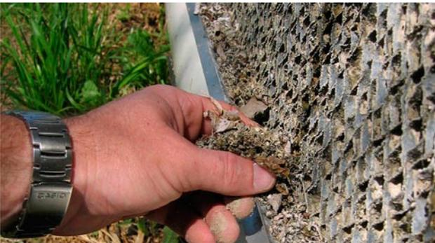
Grass clippings, leaves, dirt, and other materials must not be allowed to collect on evaporative cooling pads. Buildup like this severely reduces cooling by restricting airflow through the pad. Even worse, it will stop up a filter in a matter of seconds if allowed to enter the system water storage. It pays to keep areas around houses clean and free of trash, and never to allow grass clippings or even dust to be blown toward pads.
