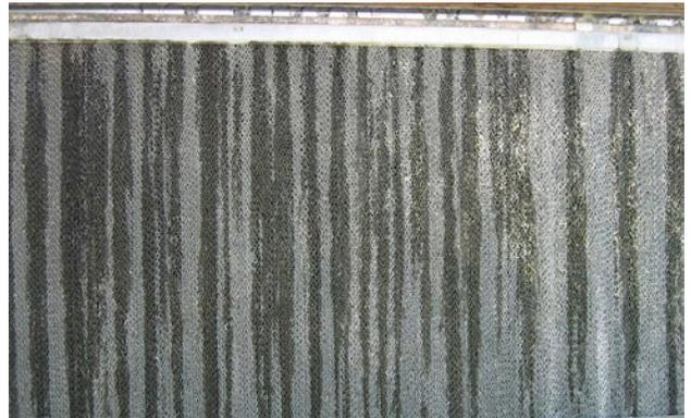
Clogged pads or headers result in dry areas on pad. Hot air coming in through dry areas causes severely reduced cooling and increased electrical costs.
