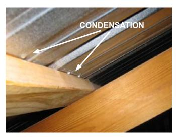
Photos above show the heavy attic condensation that can be caused by opening attic access panels. Warm and moist bird air condensing on roofing panels, as in left photo, will lead to premature rusting. Drips onto lumber, as in the photo of the purlin at right, lead to premature rotting of the roof support structure. Condensation can also cause major damage to insulation. Opening attic panels is not likely to melt enough snow off the roof to be worth taking the risk of major condensation damage.
