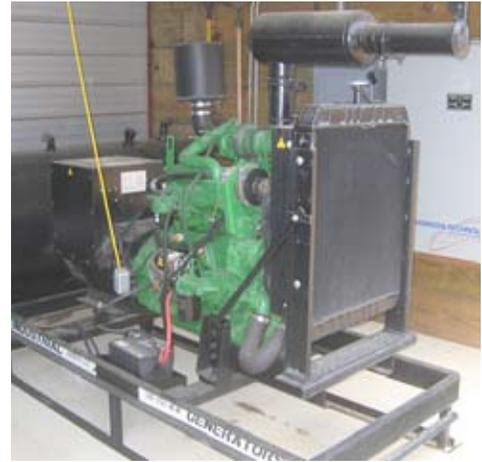
**Generator:** Generators must be fully serviced once a year and should be exercised weekly for at least an hour, actually transferring power and running the farm to ensure they can handle the full hot weather electrical load of the entire farm for as long as needed. Power outages typically last for only a few minutes, but at times can last for days.
