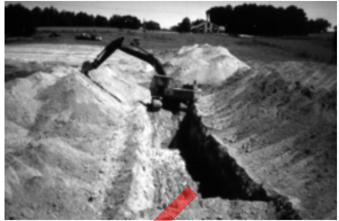
Figure 13. Excavation of cutoff trench below base of pond dam
