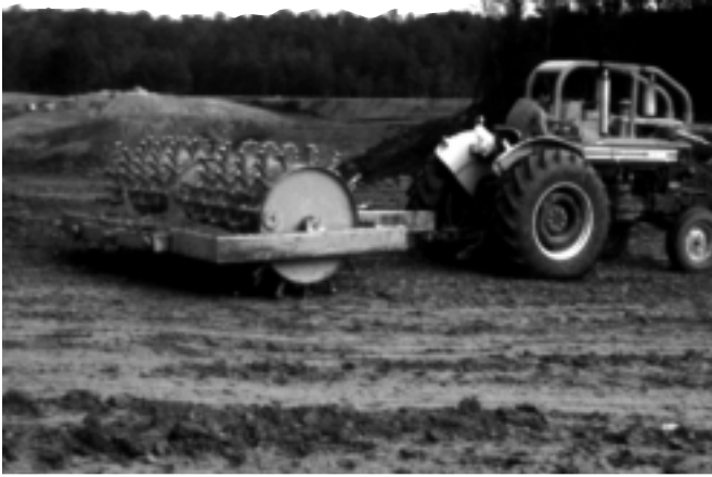
Figure 14. Using sheep's foot roller to compact earthfill
