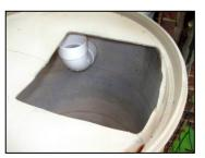
barrel installation. Drill or cut the hole to the desired size based on the pipe size being used. For 3" S&D PVC pipe use a 3 ¼" lockset type drill bit (like the ones used to drill a hole for a door knob but somewhat larger).
