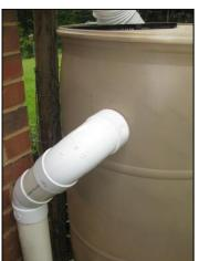
barrel in the position you wish to divert the overflow water. Make certain it does not obstruct the aquatic plant basket placement. The best location for the overflow is usually near the point the original downspout was prior to the rain
