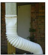
Cut the downspout (a hacksaw works well for both metal and plastic downspouts) a couple of feet above the top of the barrel.
